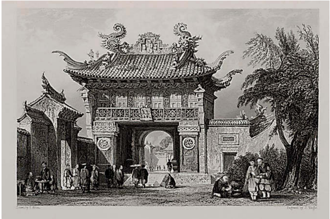
First entrance gate to the Temple of Confucius, Qinghai. Drawn by T. Allom. Engraved by J. Tingle. In 153 CE the Huandi emperor designated the Confucian temple at Qufu as a temple of the state; from then on the ruler of every dynasty always repaired a dilapidated temple after it was ruined by war or by natural disaster. BEINECKE RARE BOOK AND MANUSCRIPT LIBRARY, YALE UNIVERSITY.
