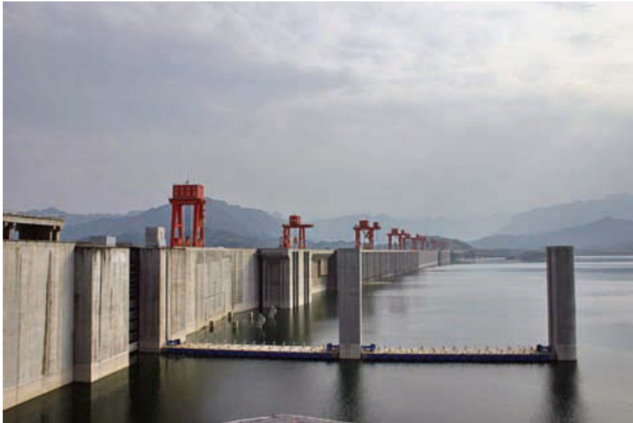
A view of the Three Gorges Dam, the world's largest feat of engineering, which will supply China with much-needed hydroelectric power when fully operational in 2009.
